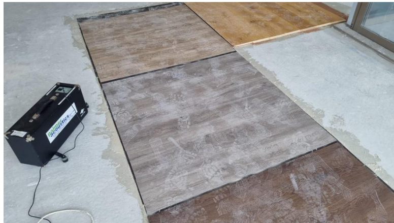
Figure 6: Test #6 – Concrete Slab
